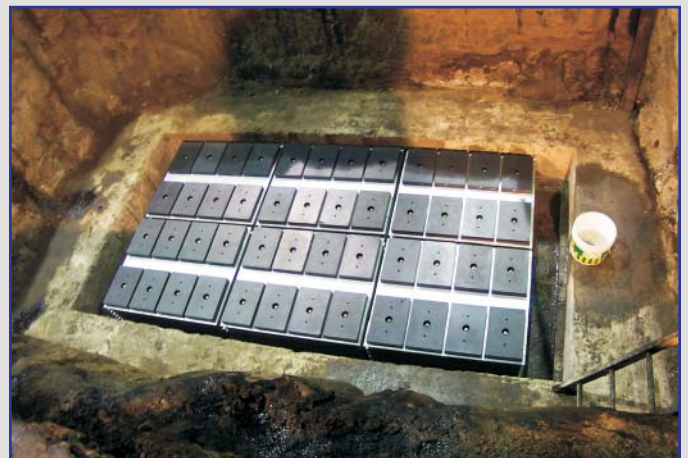
Elements quickly installed and arranged in pit.
