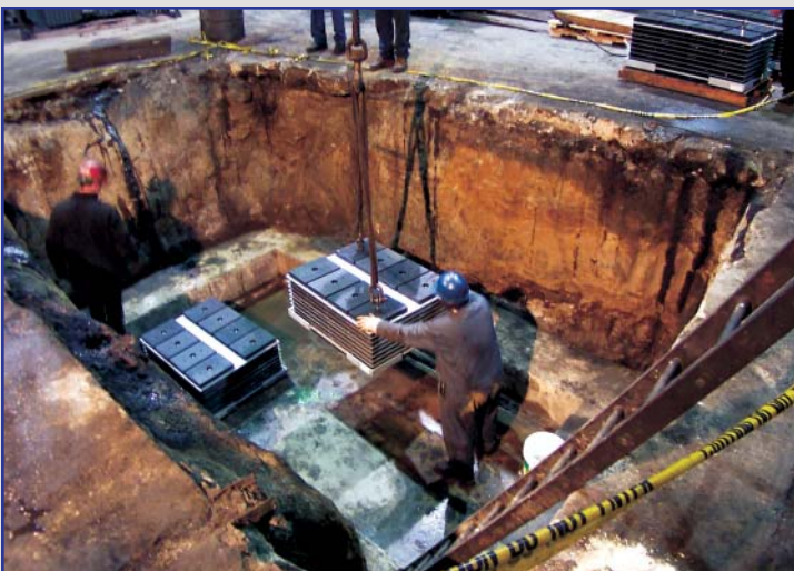
MRM Isolation Elements being lowered into a pit.
