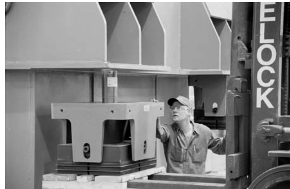
Isolators being lifted into place.
