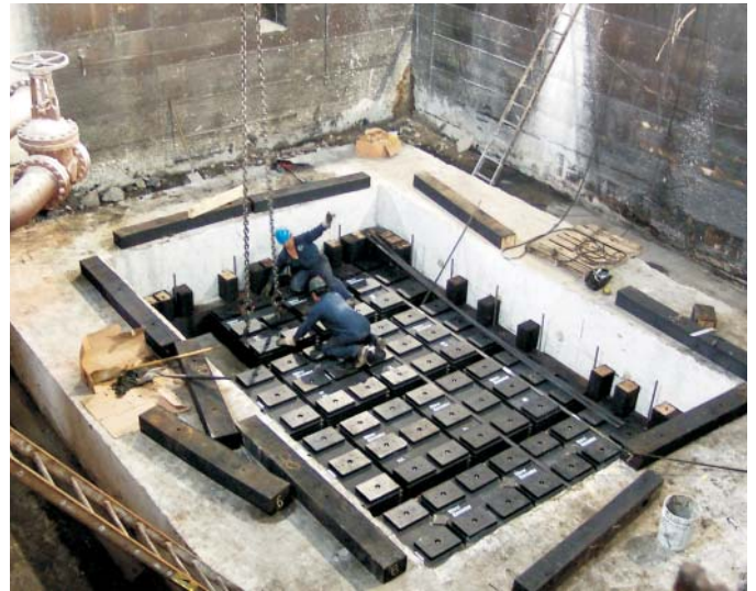
MRM Isolation Elements being placed into pit
