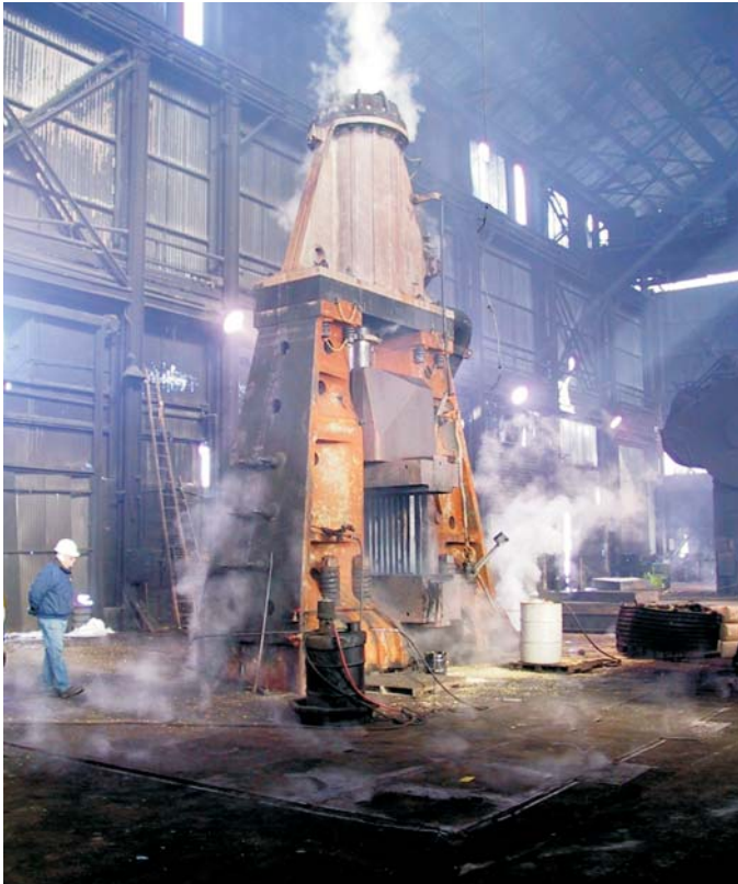
Installation of a 50,000 lb. Erie Steam Hammer Complete!
