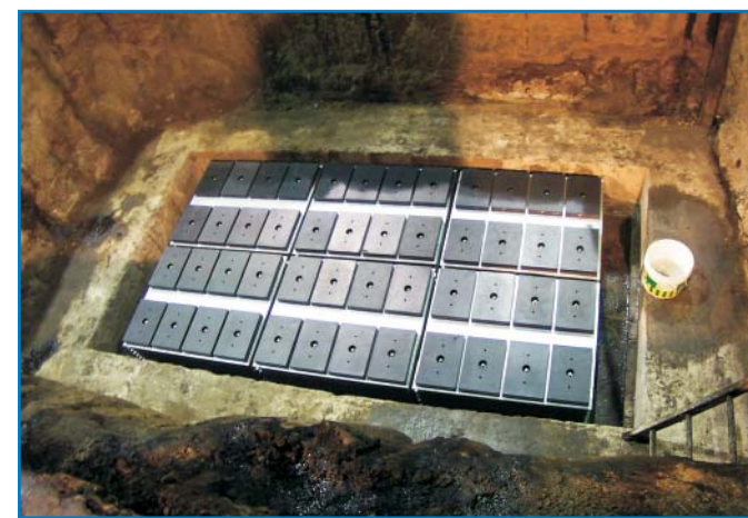
Elements quickly installed and arranged in pit.
